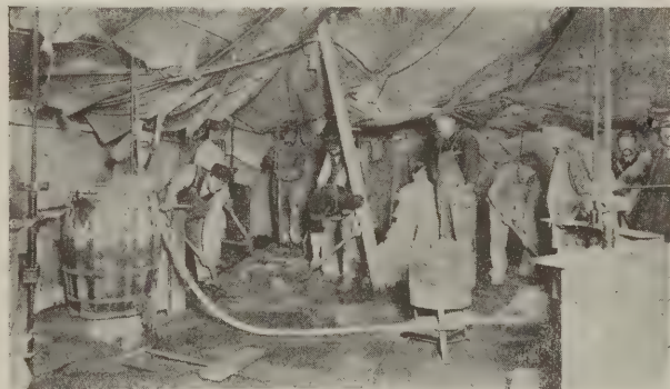
Working Under Cover
